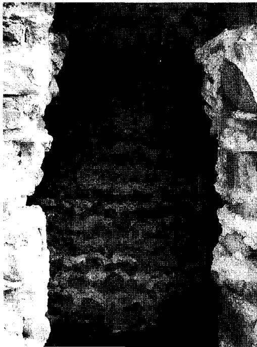
Figure 3 Detail of a niche excavated inside the town walls of Cittadella. The internal leaf is different from the external ones. It is an «opus concretum», made of regular alternate layers of pebbles with brick pieces and thick mortar beds
