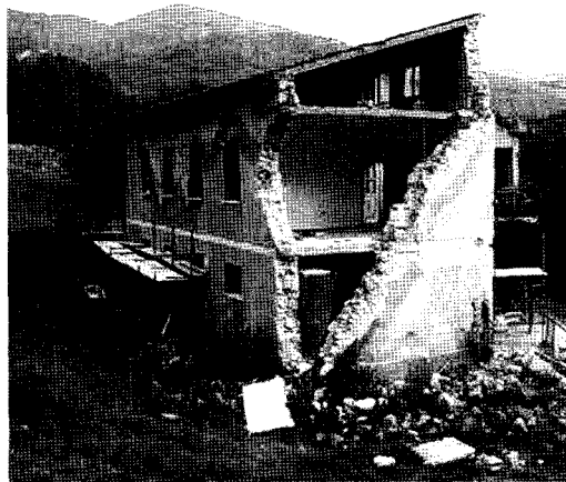
Figure 5 Global overturning of a stone masonry wall after the Umbria-Marche earthquake (Italy, 1997)
